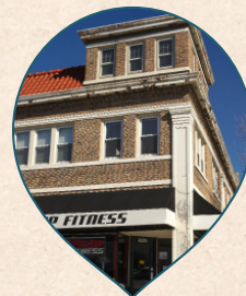
WAUWATOSA ARCADE BUILDING
